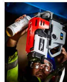
Endurance+ spray drilling upside down
